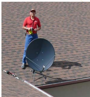
Installing satellite system in Boseman, MT conference office.
